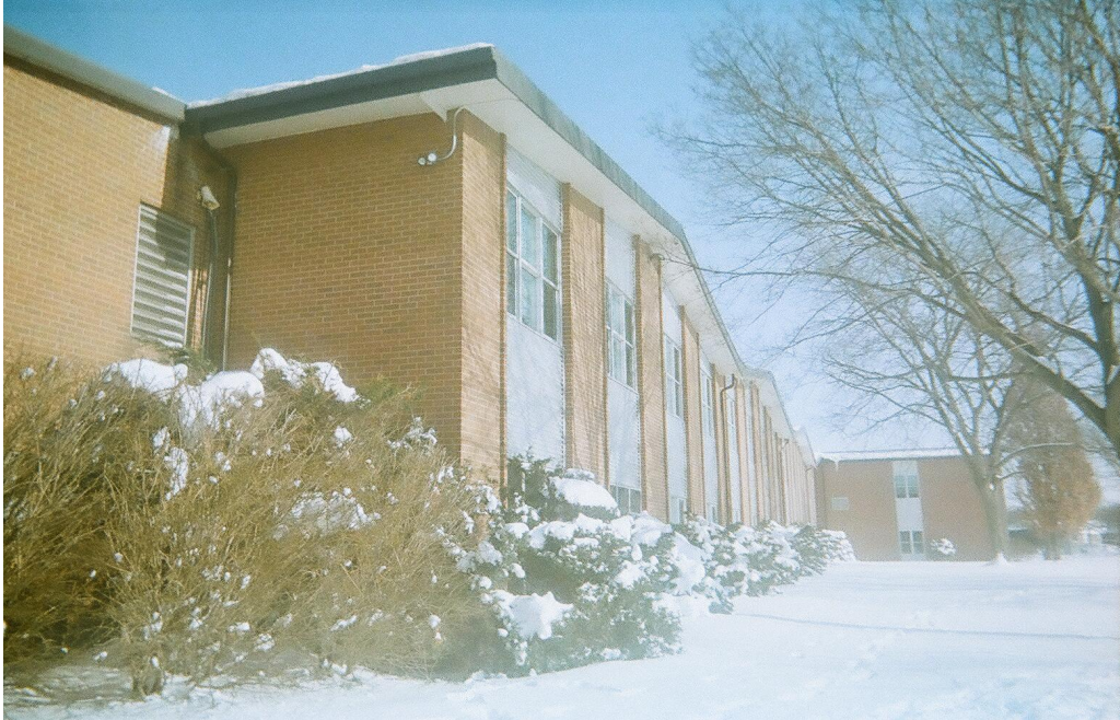
Figure 5. Student photograph: The Front of School X
